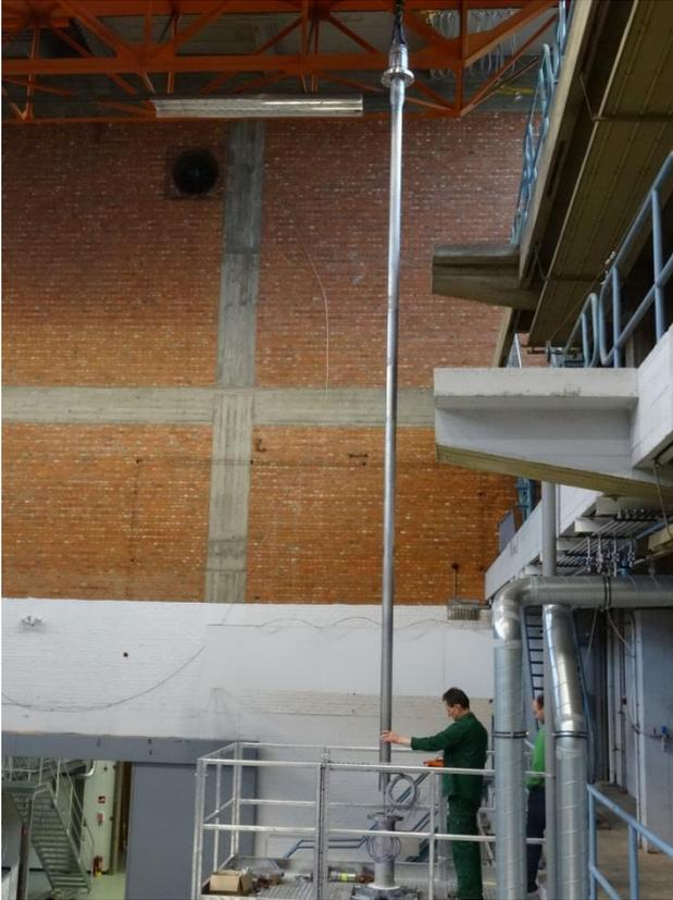
Fig. 2. CR assembly being mounted into the COMPLIT facility
